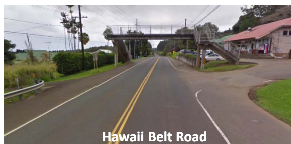
Existing pedestrian bridge, looking south
