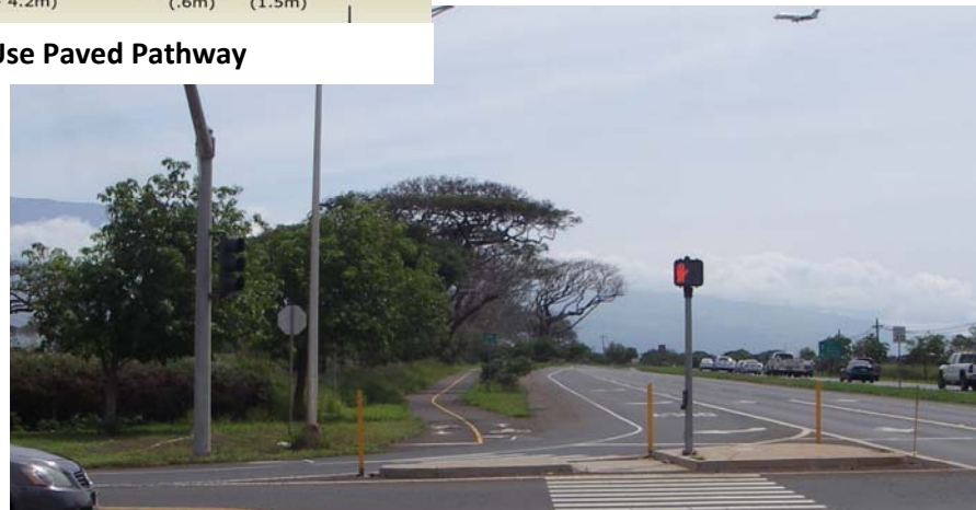
Shared use path, parallel to Mokulele Highway in Kahului, is designed to serve many types of users.
