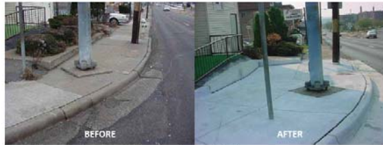
Figure 3.5 Expanding sidewalk provided space for curb ramp and landing
